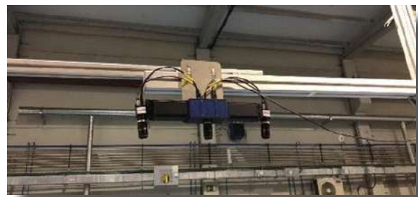
Figure 8. Stereovision cameras for identification of reinforcements and supports.
