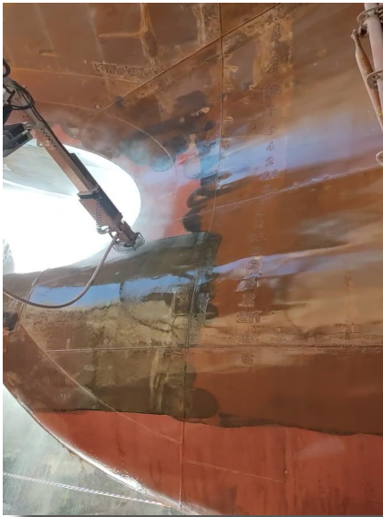
FALCH Multiworker working on flat bottom and propulsion shaft area.
