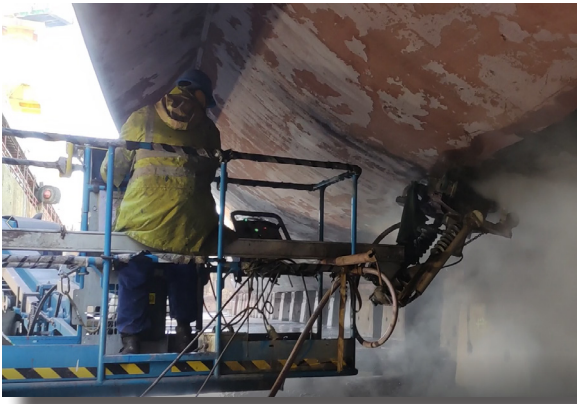
Liftworker FALCH working on bilge
