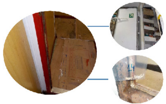
Figure 2: asbestos door joints
