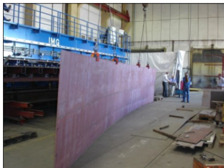
Figure 2. First 12m panel welded on the facilities of AKER YARDS Rostock in 2005.
