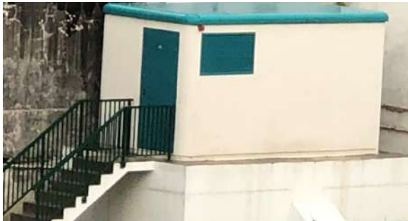
Figure 4. New disconnectors center with new 15 kV power supply.
