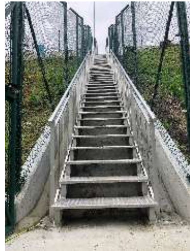
Figure 5. new access ladder.
